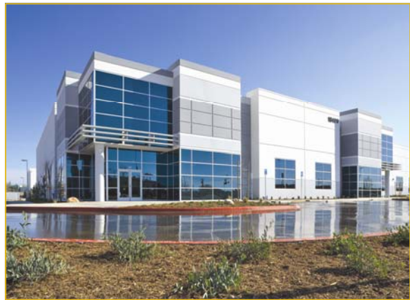
Large distribution facility at Southern California Logistics Airport
