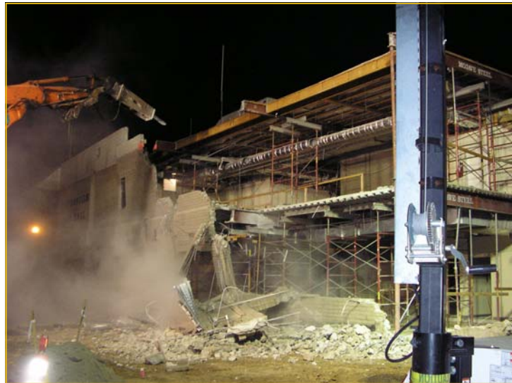
Demolition of a portion of City Hall
