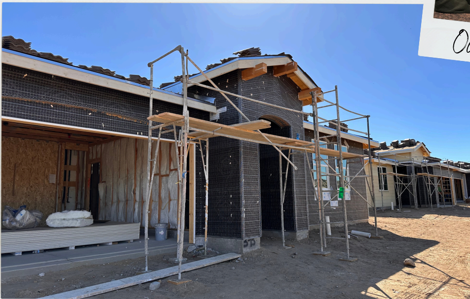
Ongoing exterior work on a tract home within a residential development.
