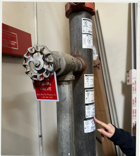
Inspection tags reviewed to confirm required inspections have been completed.
