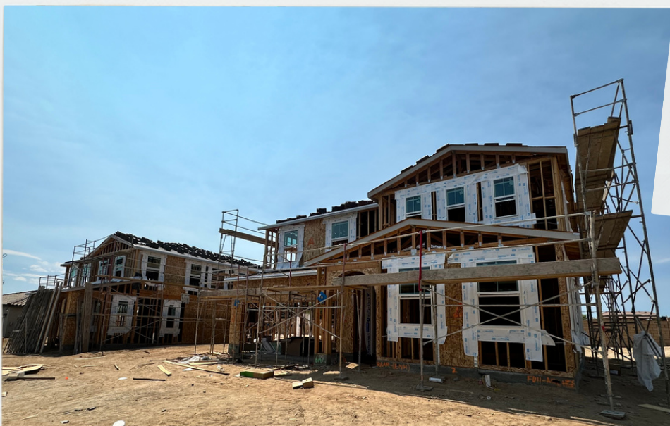
Ongoing work on a tract home within a residential development.
